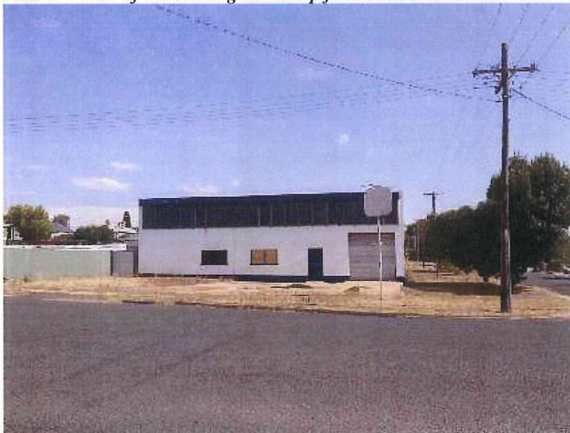
Plate 1 – View of the existing workshop from Neill Street
